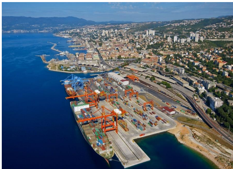
Slika 16: Adriatic Gate Container Terminal
